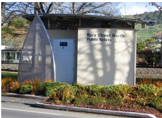
Rora Street North Public Toilets
