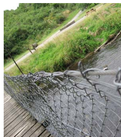
Mangaokewa Reserve Bridge
