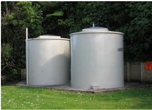
Mokau Boat Ramp Toilet
